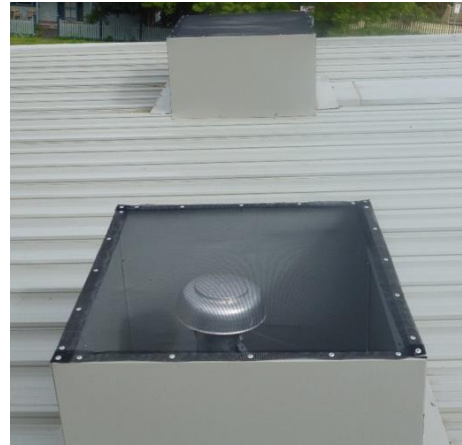
Figure 5 – Ember protection roof vents
