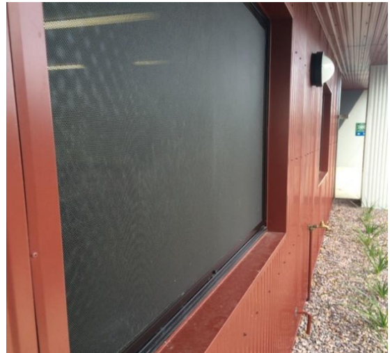
Figure 6 – Window with mesh screen protection
