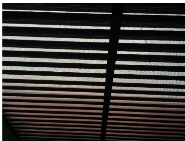
Figure 12 – Vented plant room with ember guard
