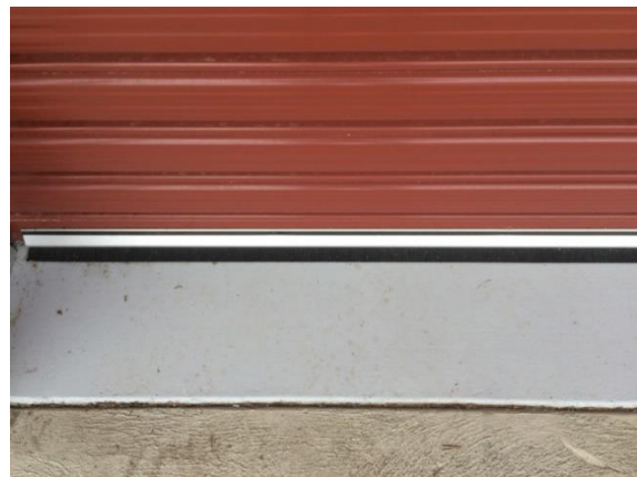
Figure 10 – Seal at base of roller door
