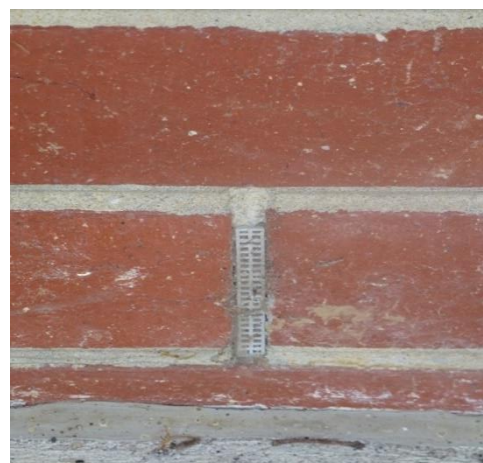
Figure 1 – Weep hole protection
