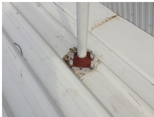
Figure 2 – Penetration seal
