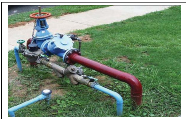
FIGURE 1 - RANGE OF TYPICAL BACKFLOW PREVENTION DEVICES
