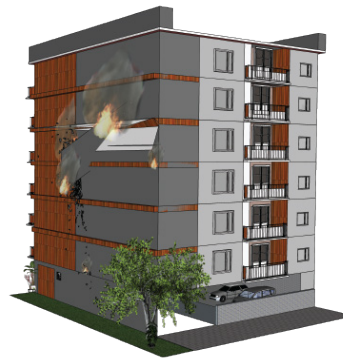
Example of ignited combustible cladding on apartment building
