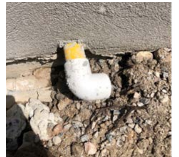
Non-compliant plastic gas pipework material used above ground.
