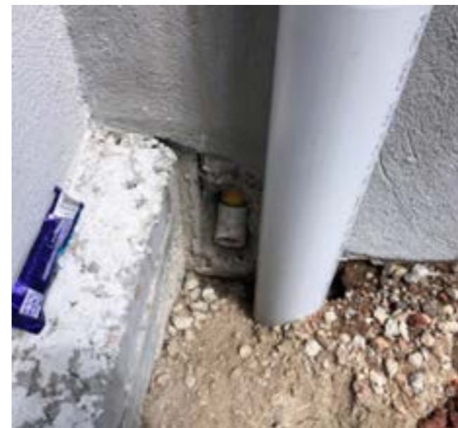
Non-compliant plastic gas pipework material used above ground.
