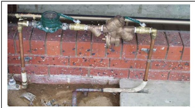
FIGURE3-REDUCEDPRESSUREZONEDEVICE- RETROFIT FOR CONTAINMENT PROTECTION
