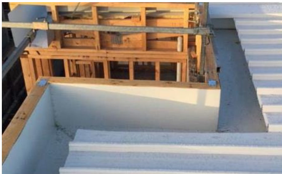
Image 1: Non-compliant box gutter (due to change of direction)
