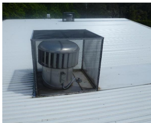
Figure 3 – Ember protect roof cowl
