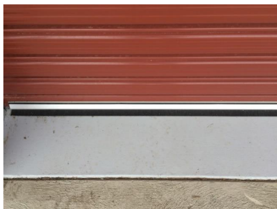
Figure 10 – Seal at base of roller door
