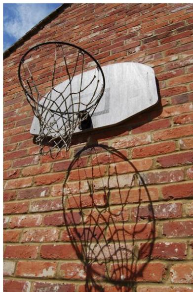
Materials can deteriorate when exposed to the elements. In addition, fixings, such as bolts and screws, can loosen with the constant banging of basketballs on the backboard and ring.
